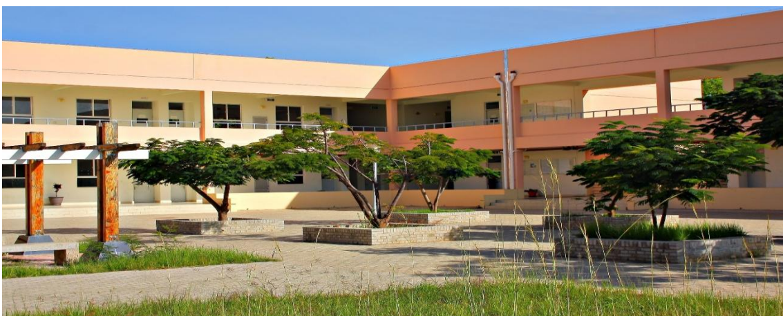
Fig. 2.2: Picture of Magistério's building
